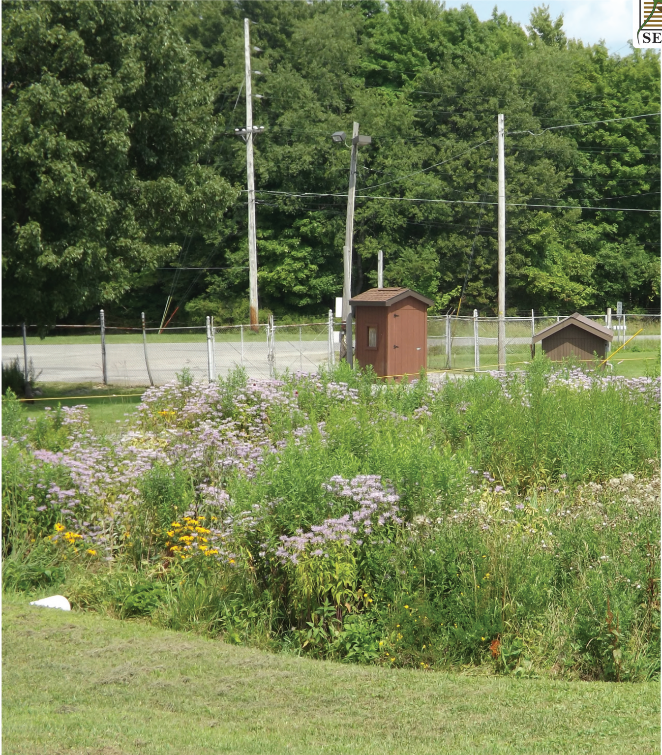
Mature rain garden at the Crawford County Fairgrounds in Meadville, Pennsylvania using ERNMX-180 Rain Garden Mix.
